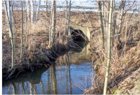
Figure 4-7: Location 3, Reshaped ditches
