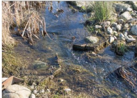
Figure 4-5: Outlet of the pond with a control structure
