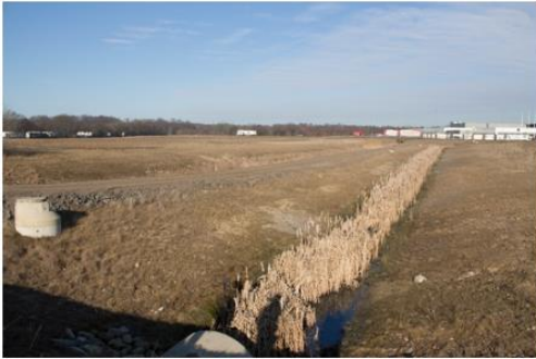
Figure 4-6: Location 2, two-stage ditch
