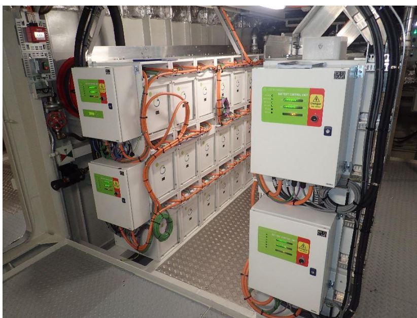
Figure 28 Example of battery installation on a passenger ferry (source: SSPA/Västtrafik)
