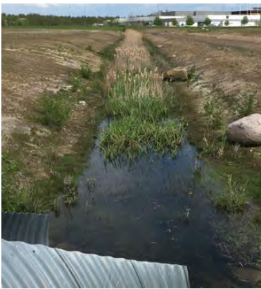
Figure 2.3.2. The two-stage channels design was constructed in 2015. The lack of shading has led to a dense in-channel vegetation.
