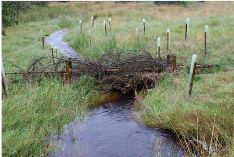
Figure 2.4.4: Engineered log structures on the Middle Burn, August 2016
