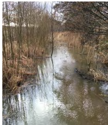
Figure 2.3.3. This stretch was constructed in 2002. It is only partially shaded. In-channel vegetation has led to heavy sedimentation. It lacks sinuosity and has no real riffle-pool sections.
