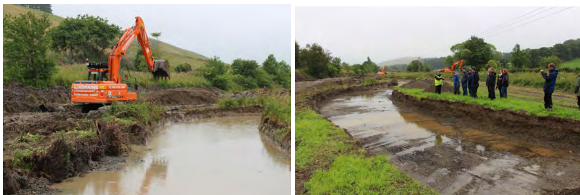
Figure 2.4.2: Remeandering the river channel at Milkiston, in 2016. Left: Gravel extraction, Right: Excavating the new channel, witnessed by some of the team-members from Work Package 4.
