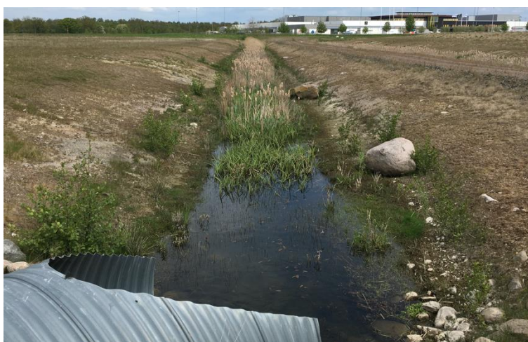
Figure 4 Study-site 2 (looking upstream), a relatively young two-stage channel restored in 2015. Photos: EA International (March 2019).
