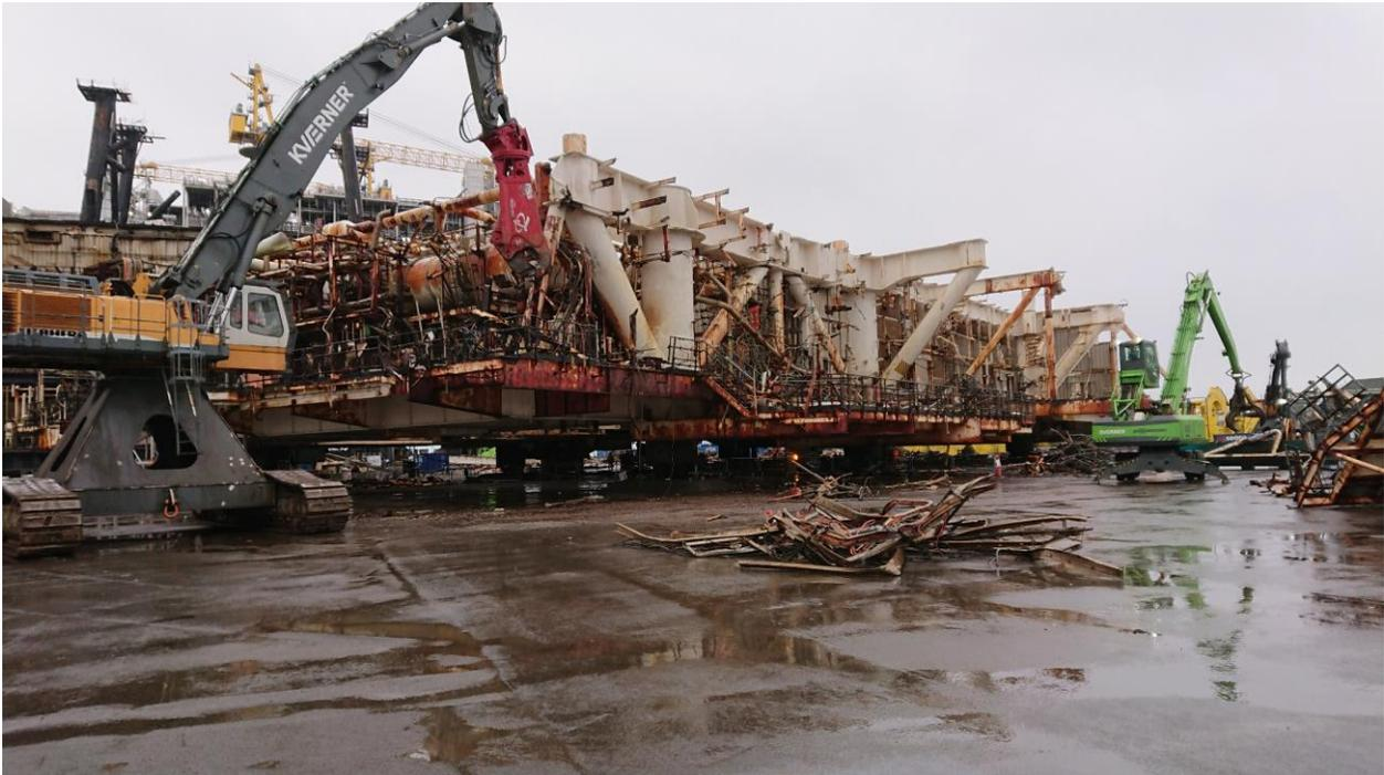
Hydraulic operated shears /scissors is used to a large extent when cutting the steel platforms into pieces. This is a very environmental friendly cutting method compared to f. ex. oxy arc /gas cutting.
