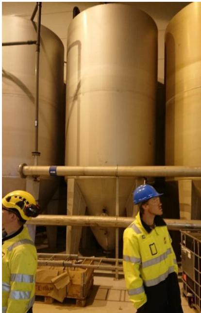
Filters for cleaning spill water.
