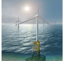
Figure 19 Fixed offshore wind turbine and foundation
