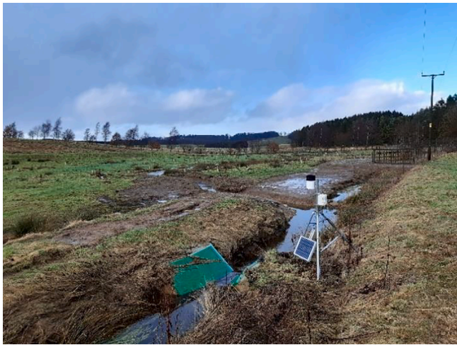
Fig. 2. Lowther Estate stream diversion by Eden Rivers Trust: channel delivers water to marsh area to the left beyond the calibrated micro-flume at Back Greenriggs.
