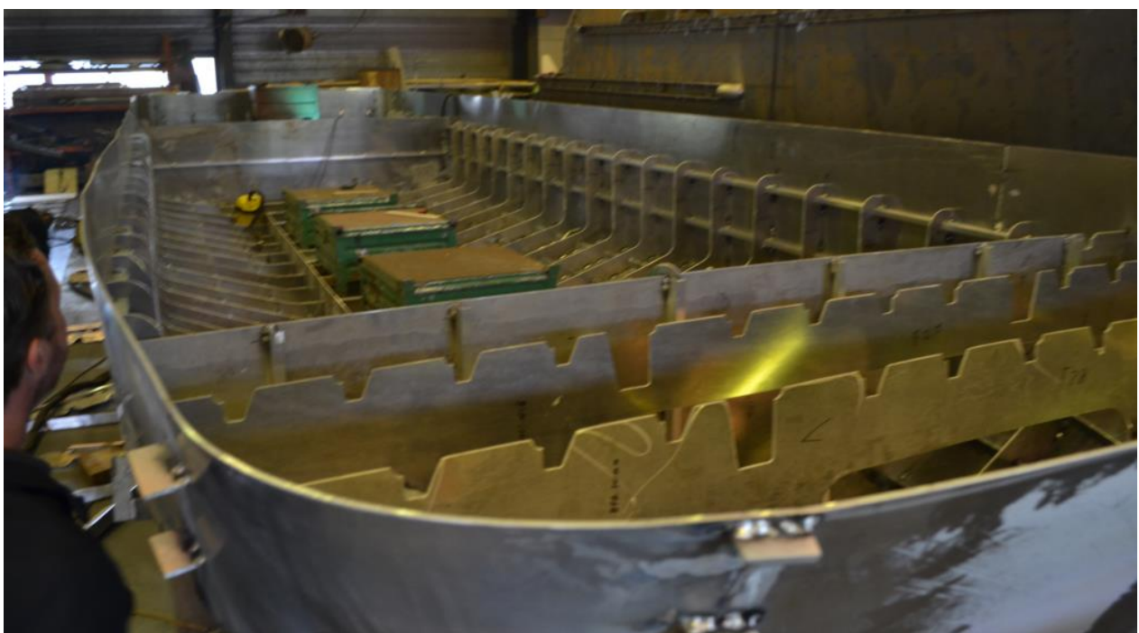
Covering the deck with alu plates
