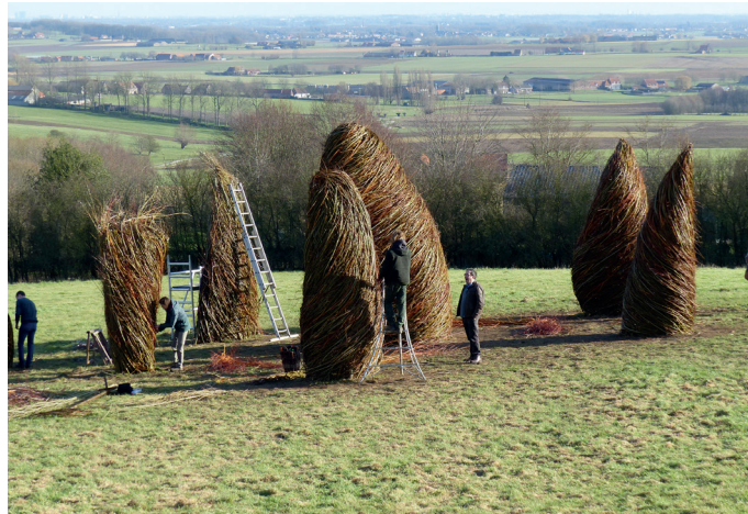
Constructing monoliths on Kemmelberg.
