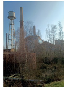
Transfo site in Zwevegem (B), setting of a living lab
