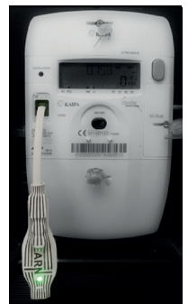
Wespark monitoring device on a smart meter
