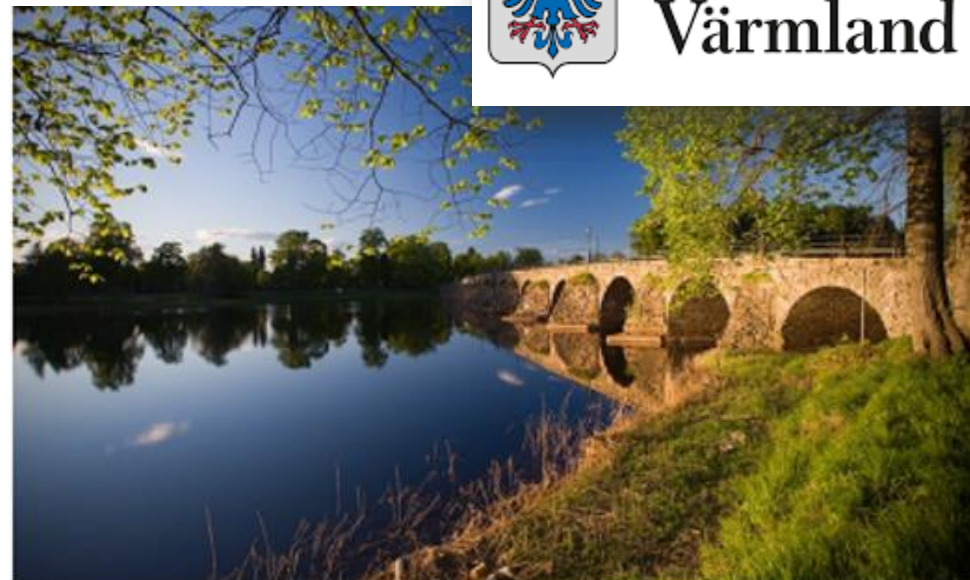
The Old Stone Bridge in Karlstad
