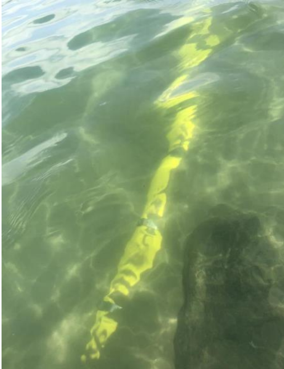
Figures 4-7. USA Block Island Wind Farm exposed cable, source [TheBlockIslandTimes, 2018]
