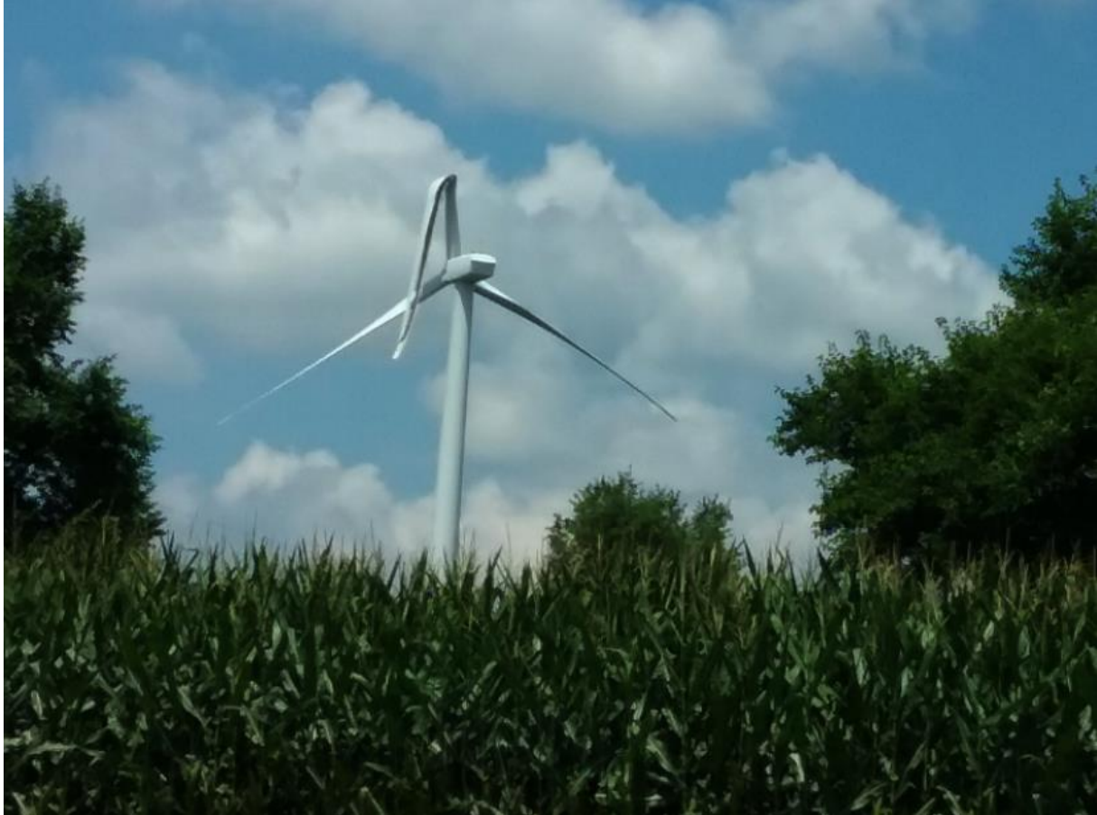
Figure 4-6. USA Iowa wind turbine blade bent, source [Times-Republican, 2018]
