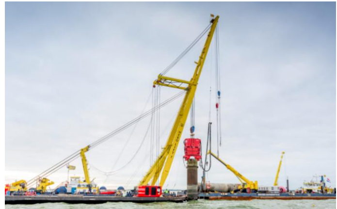
Fig. 17 Decommissioning of Lely offshore wind farm foundations, from [44]
