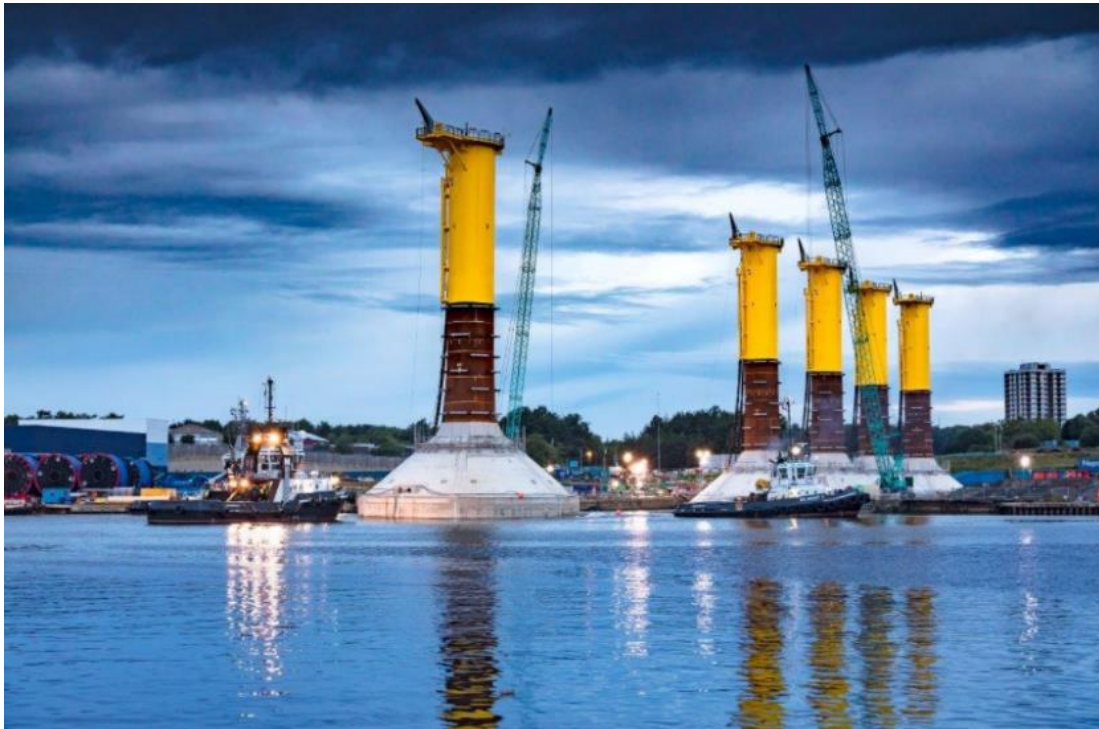
Fig. 2 gravity base foundation (GBF) for Blyth offshore wind farm, from [19]
